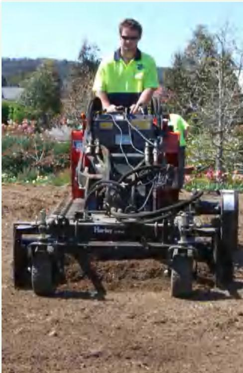
**Preparation and cultivation of the site subgrade is important to be carried out prior to installation of final topsoil.**
